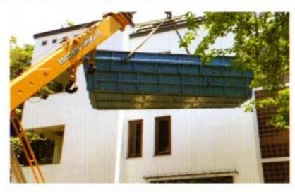
2. Placing the pool with the help of Crane at site.
