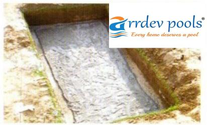
Preparation of Ground after excavation with PCC/RCC on the floor before placing the swimming pool.
