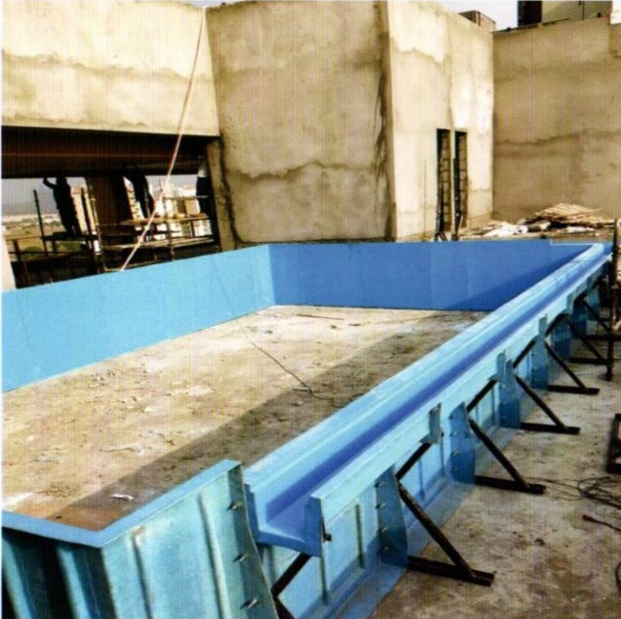
1. Step : Panels erecting
