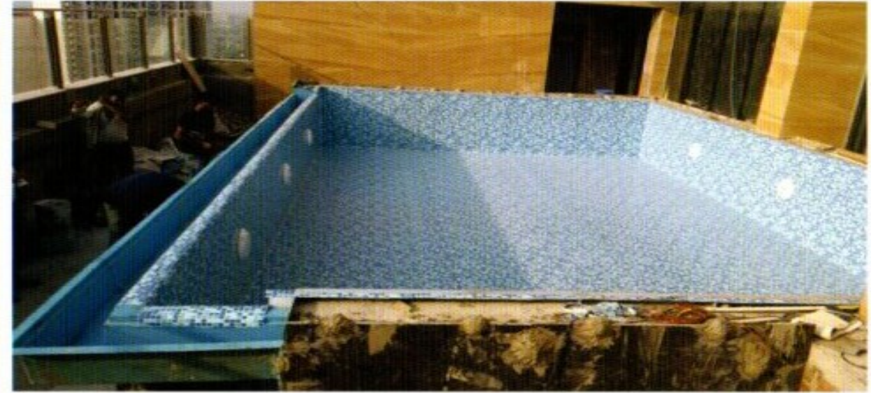
2. Pasting of Liner and Under water lights along with other fixtures.
